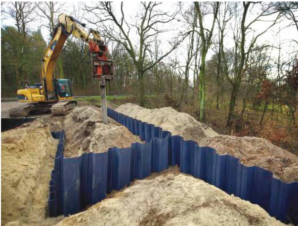
Jelcz-Laskowice, Poland. GW-610 / 9,0 Modernization of embankments.
