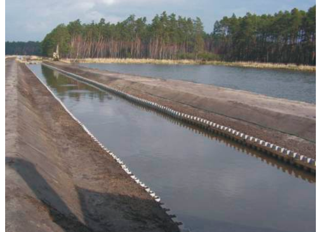
Pokój, Poland. GW-300 / 5,5 Regulation of the bed of water canal.
