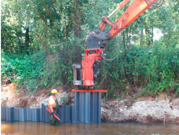
Stare Kolnie, Poland. GW 270 / 5,5 Adjustment of the bank of the river and strengthening of the waterfront.
