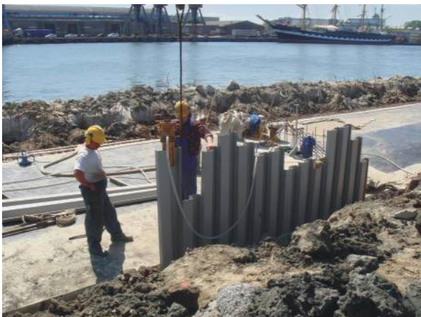
Szczecin, Poland. GW-300 / 5,5 Wharf reinforcement.
