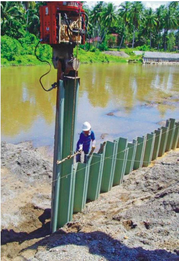
Padang, Indonesia. GW-610 / 9,0 Anti-erosion protection of the river-bed.
