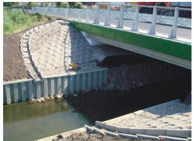
Warsaw, Poland. GW-300 / 5,5 Water culvert.
