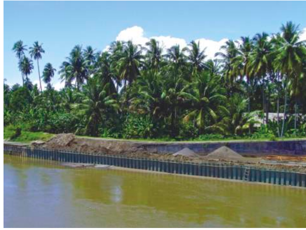
Padang, Indonesia. GW-610 / 9,0 Anti-erosion protection of the river-bed.
