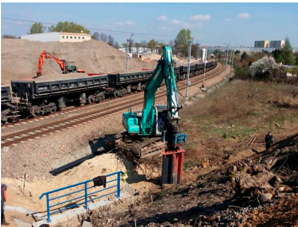
Pruszków, Poland. GW-610 / 9,0 Modernization of the railway line.
