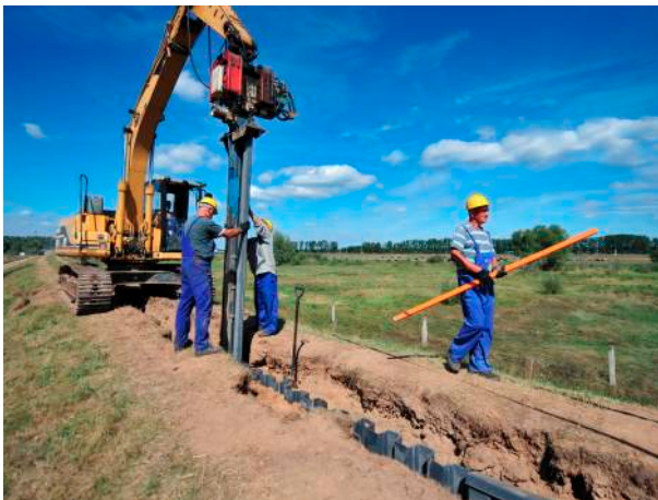
Sieradz, Poland. GW-300 / 5,5 Sealing of the flood embankment.
