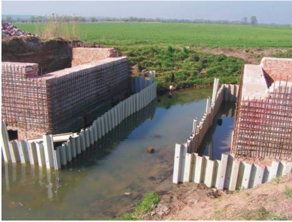
Łunawy Wielkie, Poland. GW-300 / 5,5 Securing foudation of a hydroelectric power plant.
