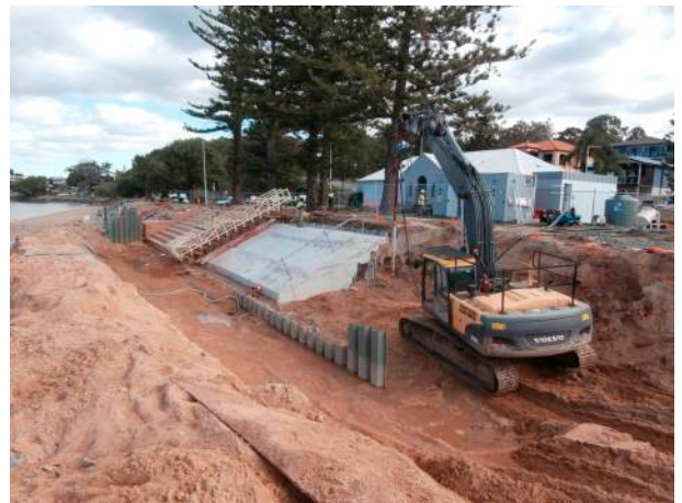
Scott's Point, Australia. GW-610 / 9,0 Protection of the seawall.
